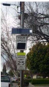
The photo taken in San Jose, California by the author illustrates the case (note the wooden utility pole located within feet of the solar-powered traffic safety device). Hundreds of thousands of these speed feedback signs are now in place across North America and few use grid power for the reasons described. Like the railroads, if IOUs thought of themselves as being in the **power selling** business, rather than in the **streetlight** business, this might not have been the case.
