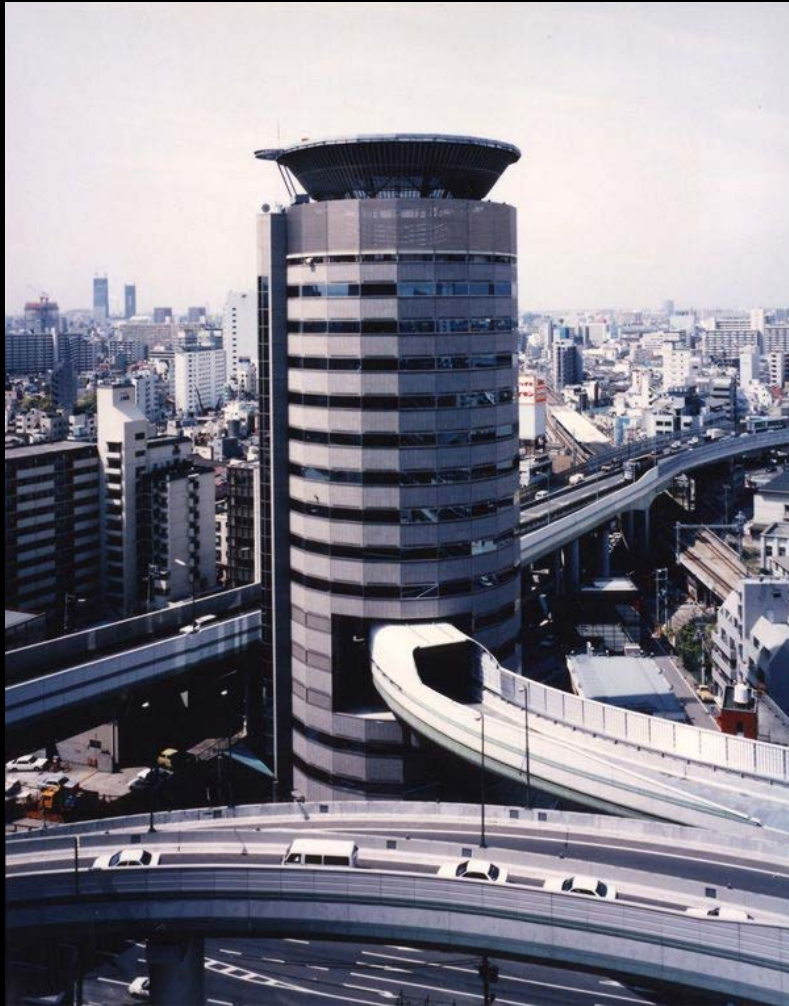
Freeway is the tenant of the 5th and 6th stories of this Japanese building
